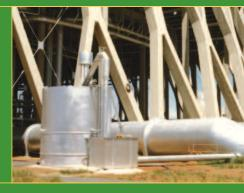
**Application**Bore-Hole water, iron, manganese and solids removal for drinking purposes
